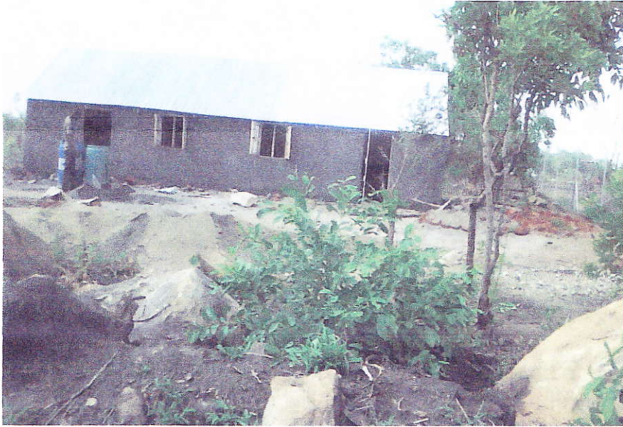
Church being built in refugee camp
